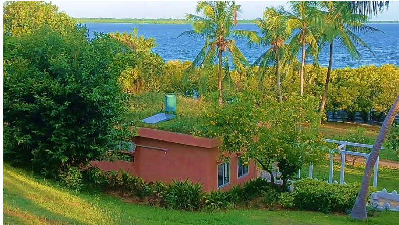
Solar hot water mounted on the green roof system
